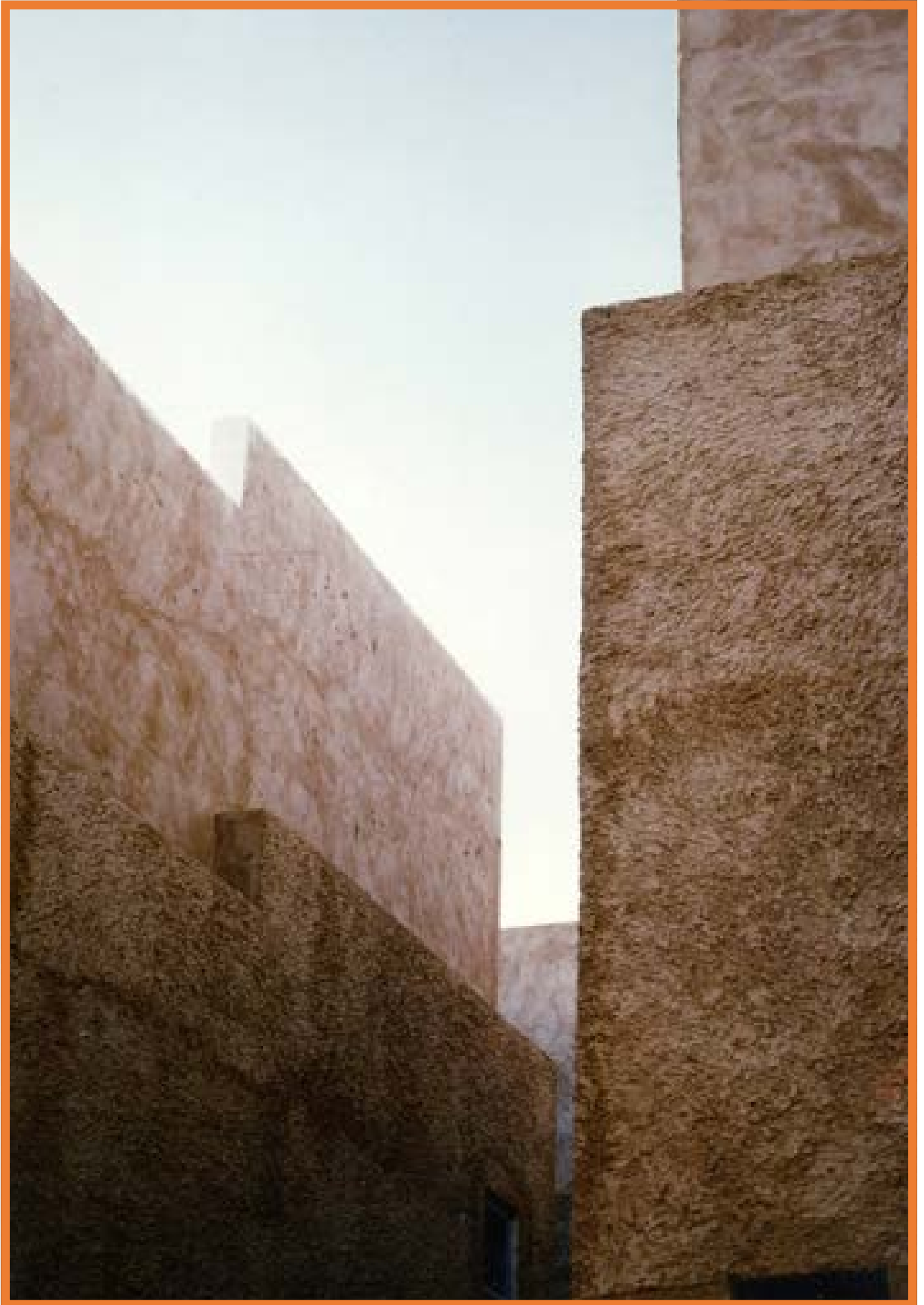
Housing Sidi Abbaz, Mzab Algeria, André Ravéreau Manuelle Roche ADAGP 1976
