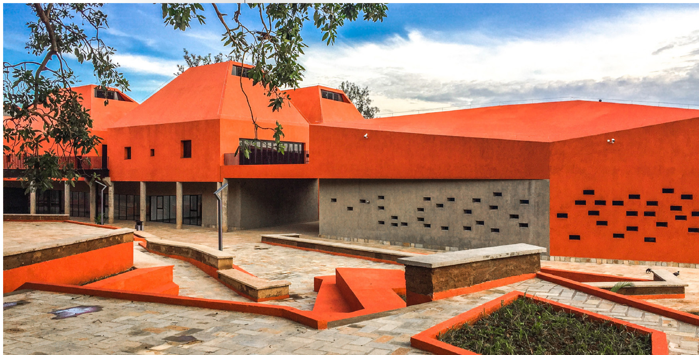
School of Architecture and Built Environment, Photo source SABE
