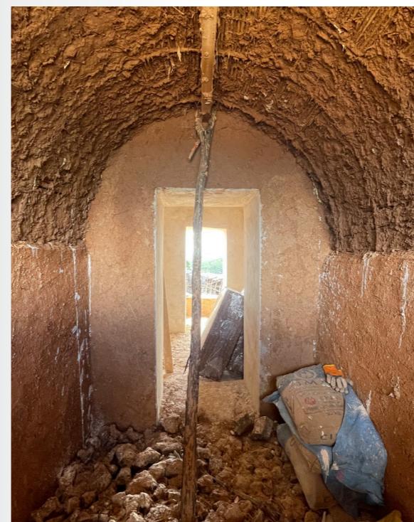
Application of straw earth layer, Photo by A&D
