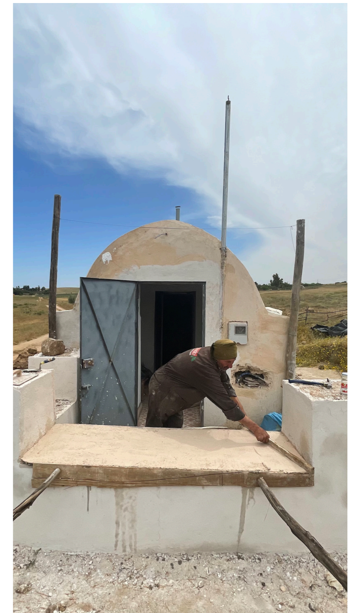
Application of sand lime coatings, Photo by A&D
