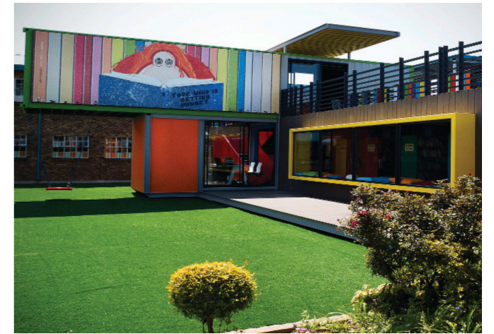
Architects of Justice, Seed library (Afrique du Sud), Courtesy of CAASI
